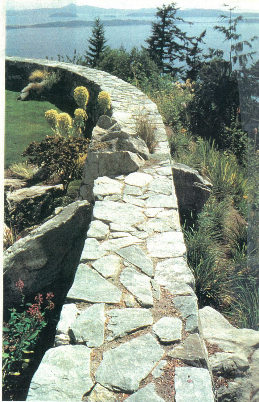
Schraven constructed these walls with stone wedging without using mortar.
