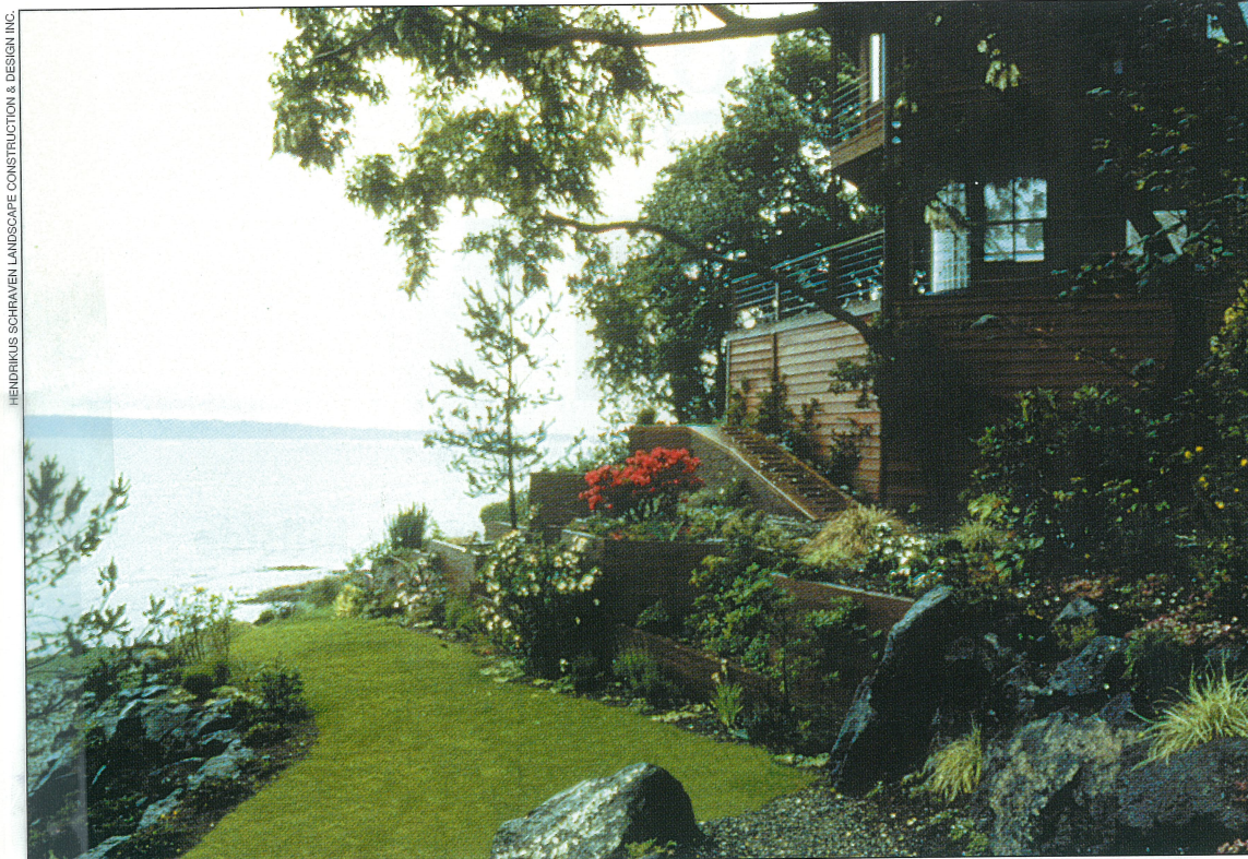
Great care was taken to protect root systems of the existing plant materials that surrounded the lower house at the base of the hillside (below). Retainers, planting beds and rock settings were used to help create a beautiful landscape (left). The interlocking 4-foot by 6-foot retainers are built with a complete drainage and irrigation system, and are filled with a light, rich, organically amended topsoil/compost blend.
