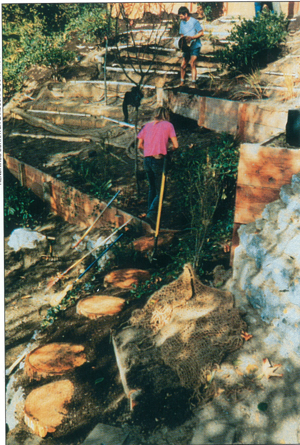
This side view from the upper hill (left) shows erosion control with use of erosion netting and dirt held firm with untreated boards that will biodegrade after vegetation root systems are well-established. Seven months later (below), the ivy ground cover has taken over, and other native plantings actively stabilize the hillside.
